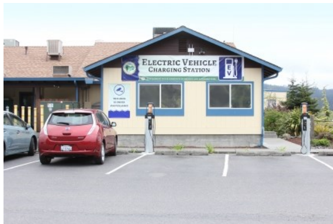
Blue Lake Rancheria: Electric vehicle charging stations in front of the Tribal Office (February, 2015) Photo Credit: Toni Ramos, Blue Lake Rancheria
