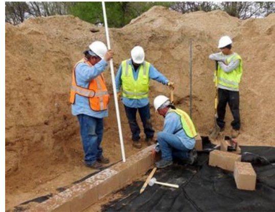
The Ohkay Owingeh workers are replacing a 60-foot span
